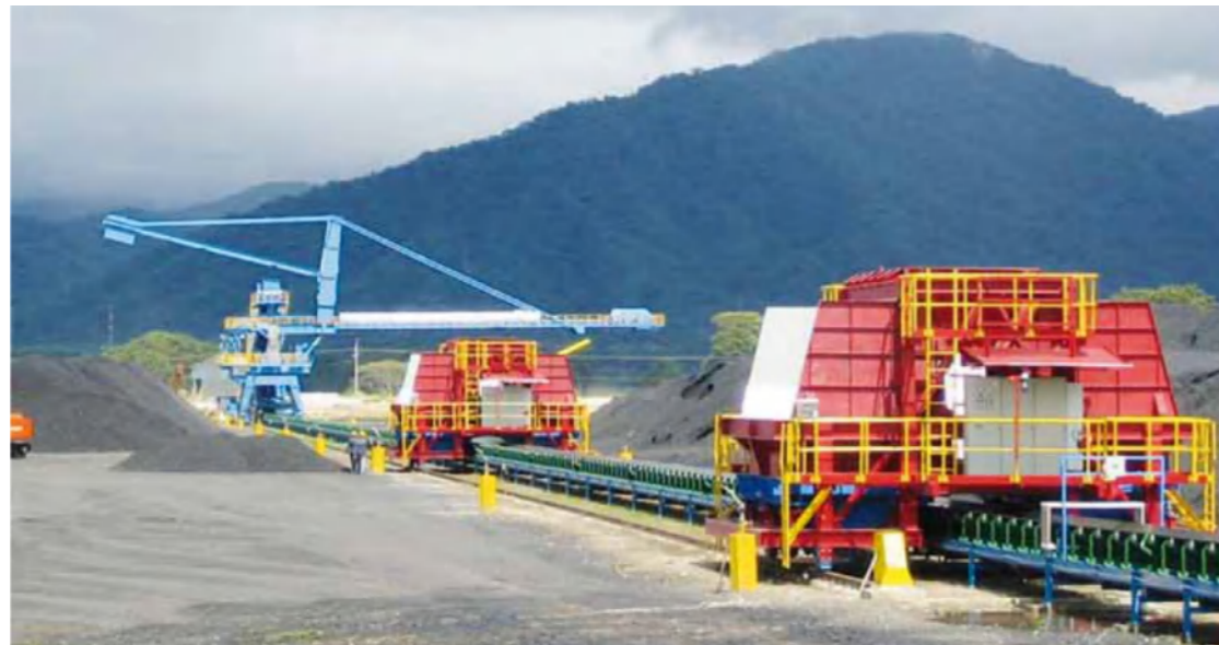
Mineral deposits conveyor
